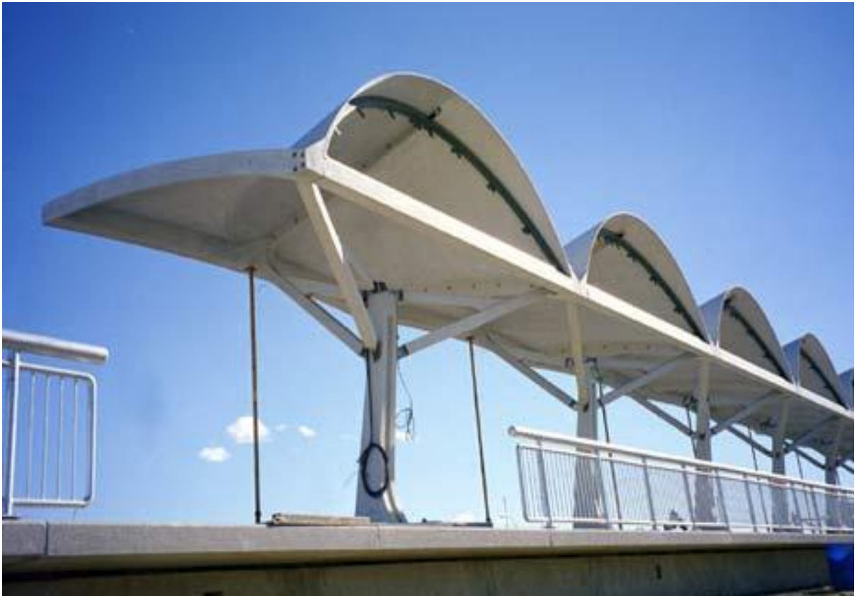
Fig 5.3 Half-canopy Light Rail Transit Station, Calgary, Canada
